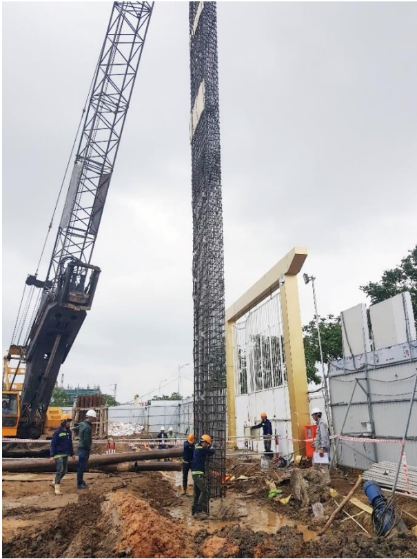
Figure 1. Barrette walls have rectangular cross-sections
